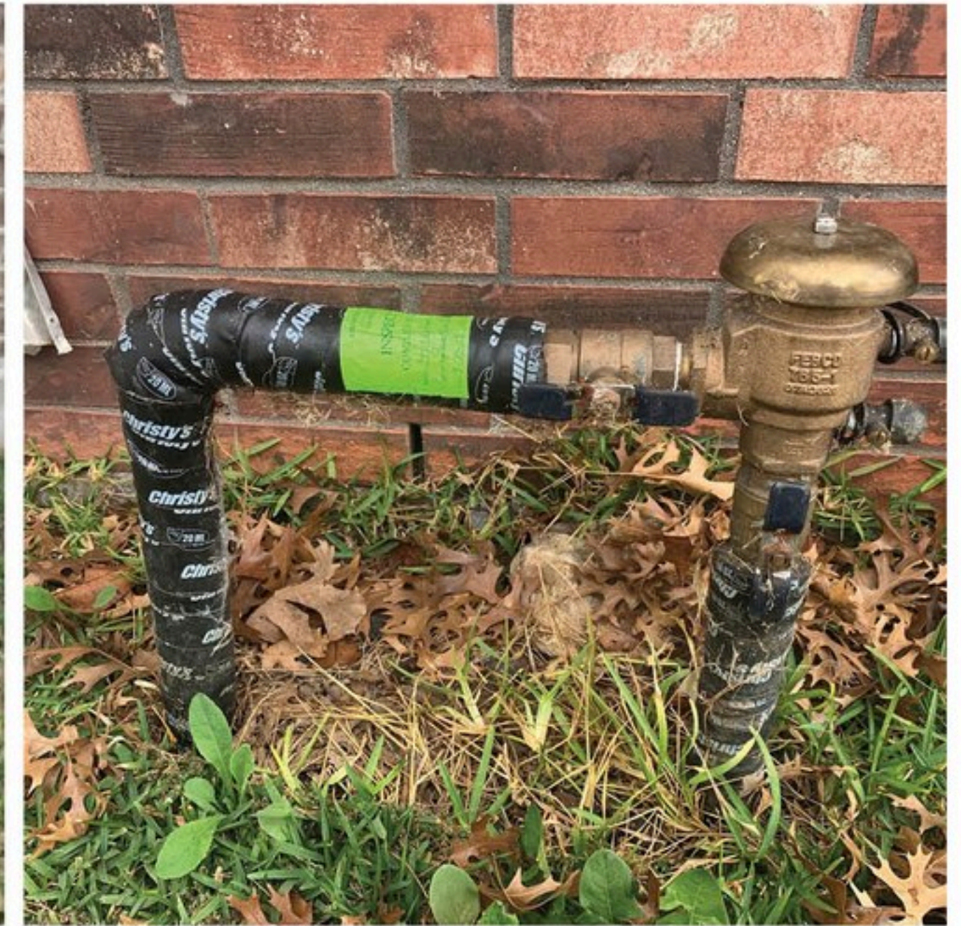
Back flow devices are required on customer services lines that have an irrigation system. Devices with no insulation (like the two above) are susceptible to freezing. An insulated covering (like the two shown below) can help protect the device.
