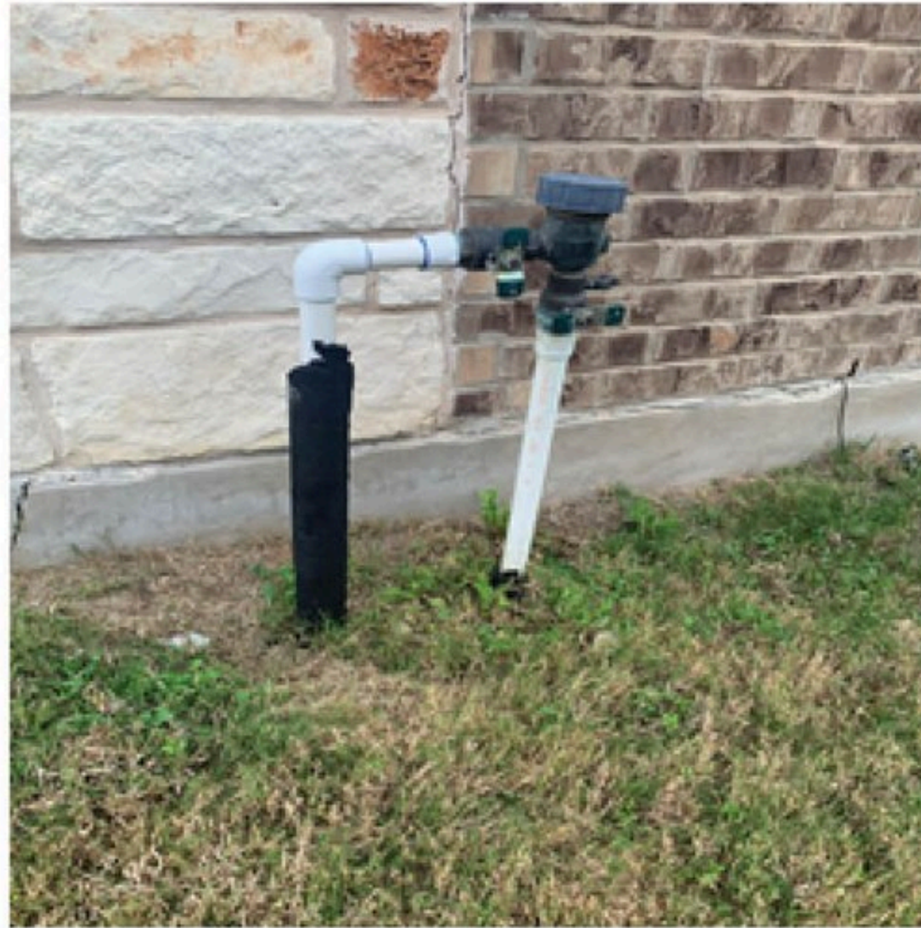
Back flow devices are required on customer services lines that have an irrigation system. Devices with no insulation (like the two above) are susceptible to freezing. An insulated covering (like the two shown below) can help protect the device.
