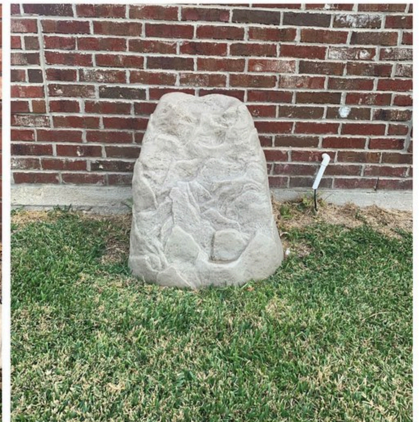
Uncovered water faucets are susceptible to freezing, so be sure to use a faucet cover, like the one shown on the right:
