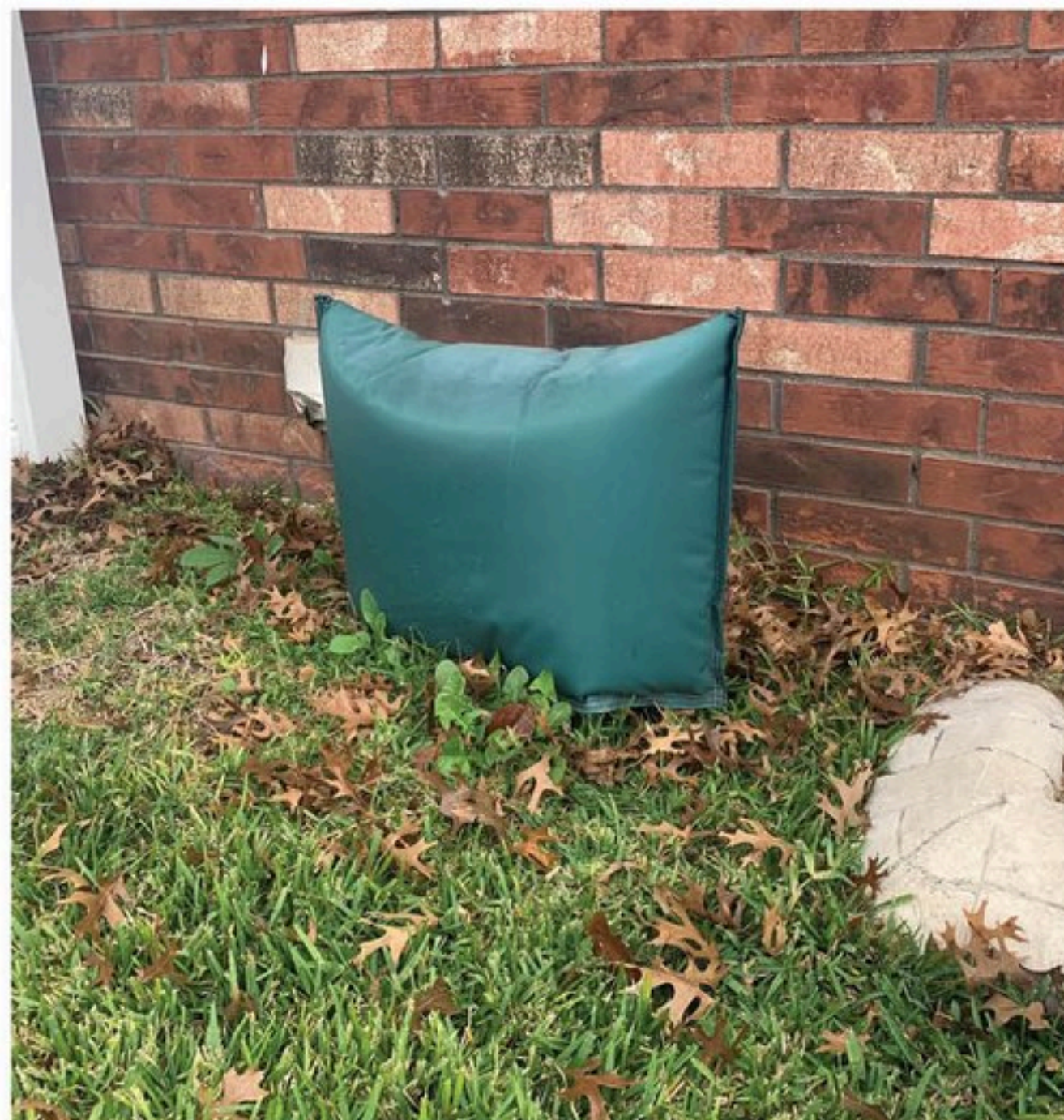
Uncovered water faucets are susceptible to freezing, so be sure to use a faucet cover, like the one shown on the right:
