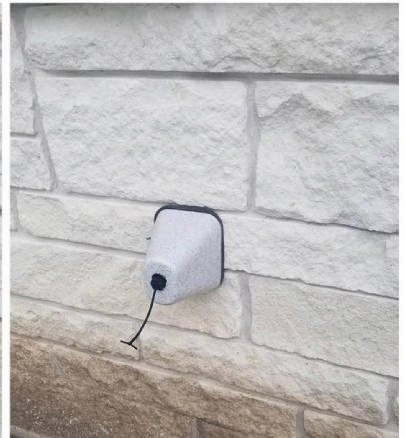
Uncovered water faucets are susceptible to freezing, so be sure to use a faucet cover, like the one shown on the right:
